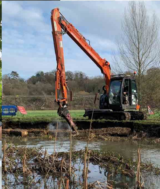
Removal of ecologically-harmful concrete revetments during restoration at Waterford Marsh in 2023.
